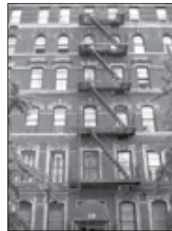
When you visit an apartment, ask the landlord where the fire exits are. Tall apartment buildings have fire escape stairs on the outside of the building. Bigstockphoto.com
